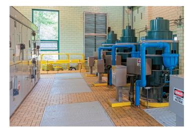
The general design of a pump station depends on different components such as power supply source, storage, pumping capacity and piping. Analyzing the hydraulic capacity of these components — by factoring in average dry weather flow and peak wet weather flow — will assist in building or retrofitting a pump station.
