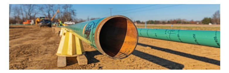
External coatings are the first line of defense for buried metal pipelines. They serve as a barrier that separates the metal from the surrounding soil or water, which, acting as electrolytes, can set off corrosive electrochemical reactions. Furthermore, contact with abrasive environments can inflict mechanical damage to buried pipelines and shorten their useful life. Selecting coatings that protect pipeline integrity are therefore critical to pipeline reliability and longevity.
