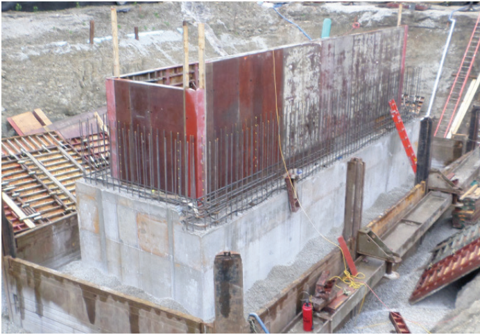
Figure 1: Construction of new West Pump Station at old West WWTP.
