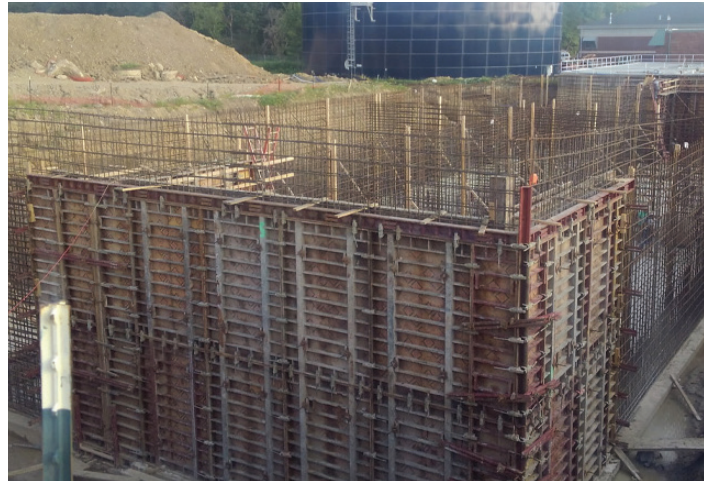
Figure 2: Construction of new aerobic digesters at Regional WWTP.
