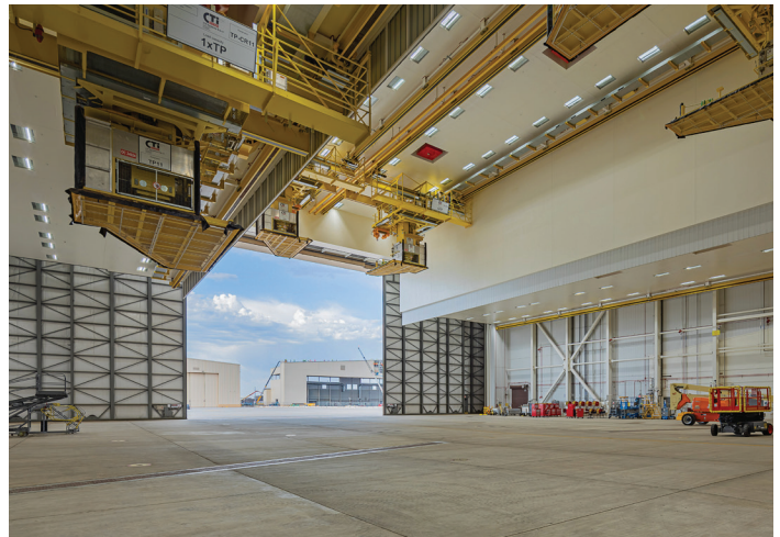
Figure 1: The innovative hangar provides the U.S. Air Force with support needed for aircraft maintenance requirements.
